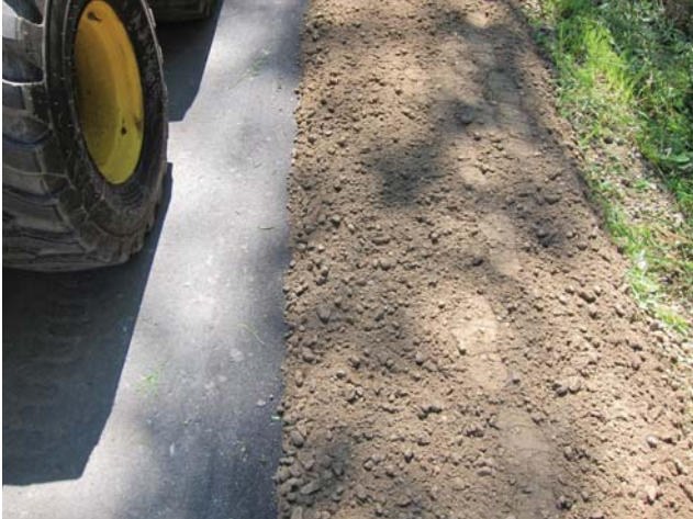
Figure 42: Ensuring Material is Above Road Surface
