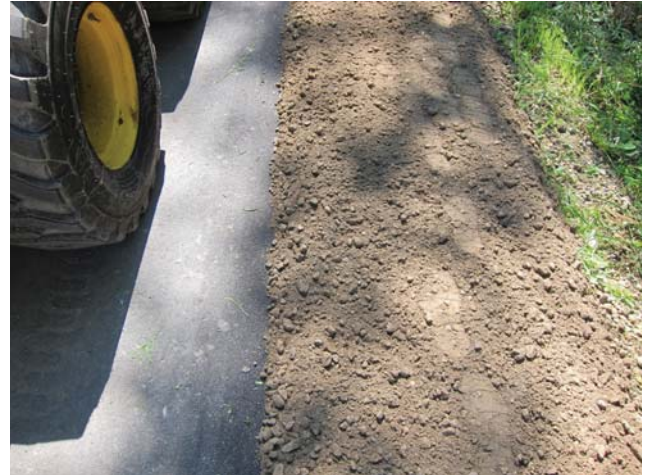
Figure 58: Ensuring Material is Above Road Surface
